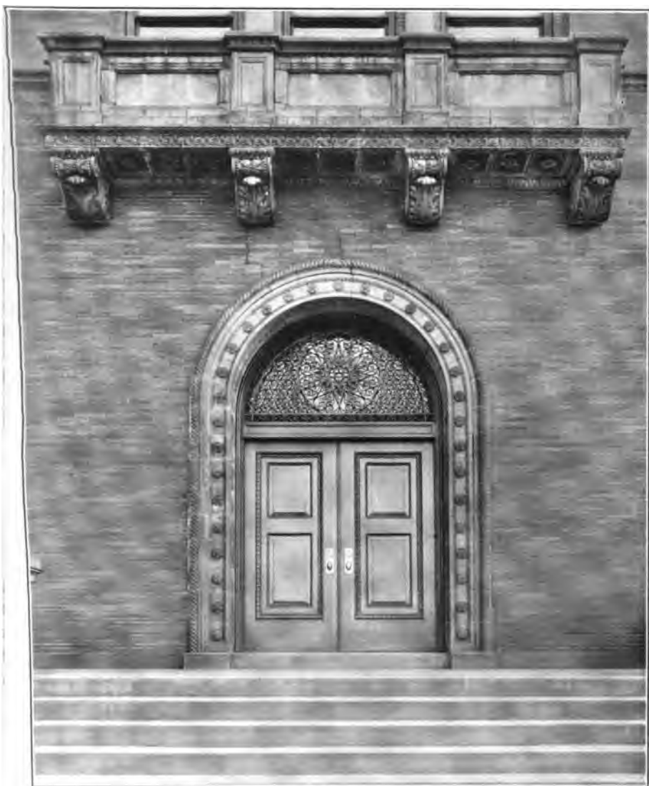
BALCONY AND ENTRANCE, CARNEGIE LIBRARY, HOMESTEAD
